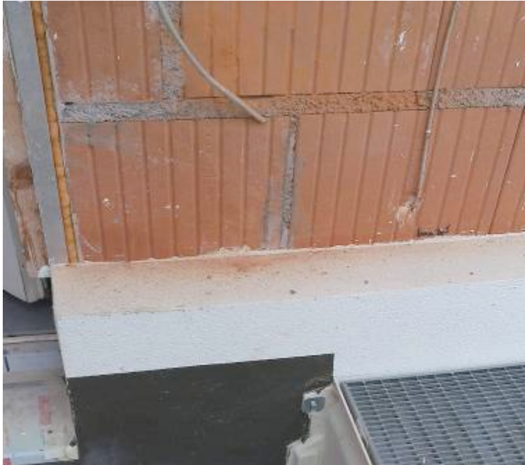
Fig 9: Perimeter insulation installed to the foundation of a new build property.
