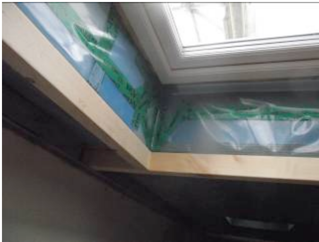
Fig 10: A well-implemented Swedish airtightness detail
