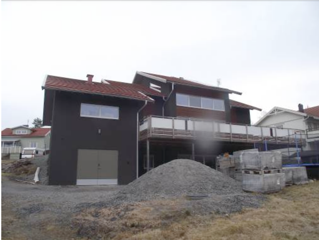
Fig 7: Rear view showing steps, staggers, glazed areas, integral garage (which is multi-storey) and balconies
