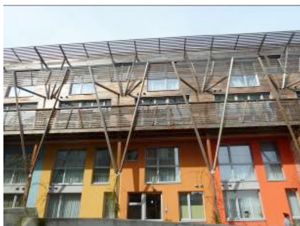
Fig 5: Typical Brussels new build - in this case a Passivhaus apartment block with a very simple structural form and solar shading
