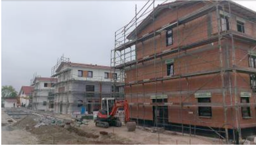
Fig 4: German clay honeycomb block (solid wall) masonry construction (rendered on the left and prior to render on the right)
