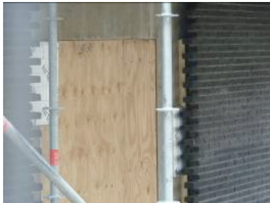
Figure 2: An opening in a Brussels apartment block showing the concrete inner leaf with masonry outer leaf
