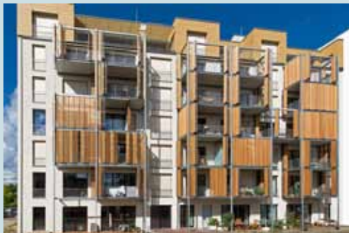
Boyden Street zero emissionbuilding Berlin Germany Deimel Oelschläger Architekten Award recipient (apartment building)
